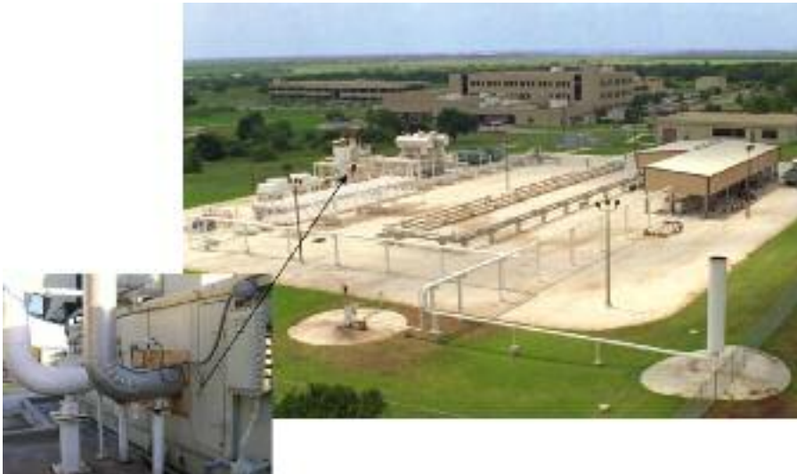
FIGURE 4.3. The metering research facility (MRF) at the Southwest Research Institute, San Antonio, Texas.
